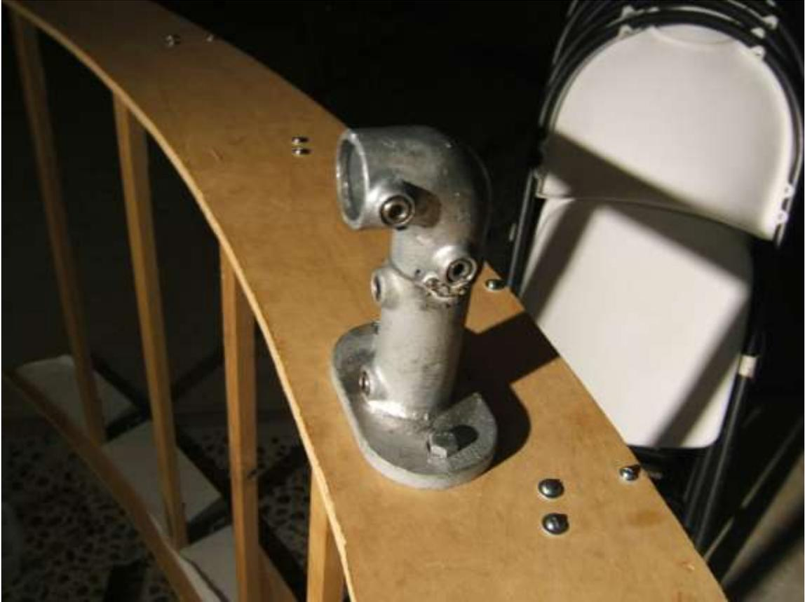
This weld connecting these two pipe fittings is essential, as there is a tremendous amount of torque at this joint and an exact 90 degree angle is essential.
