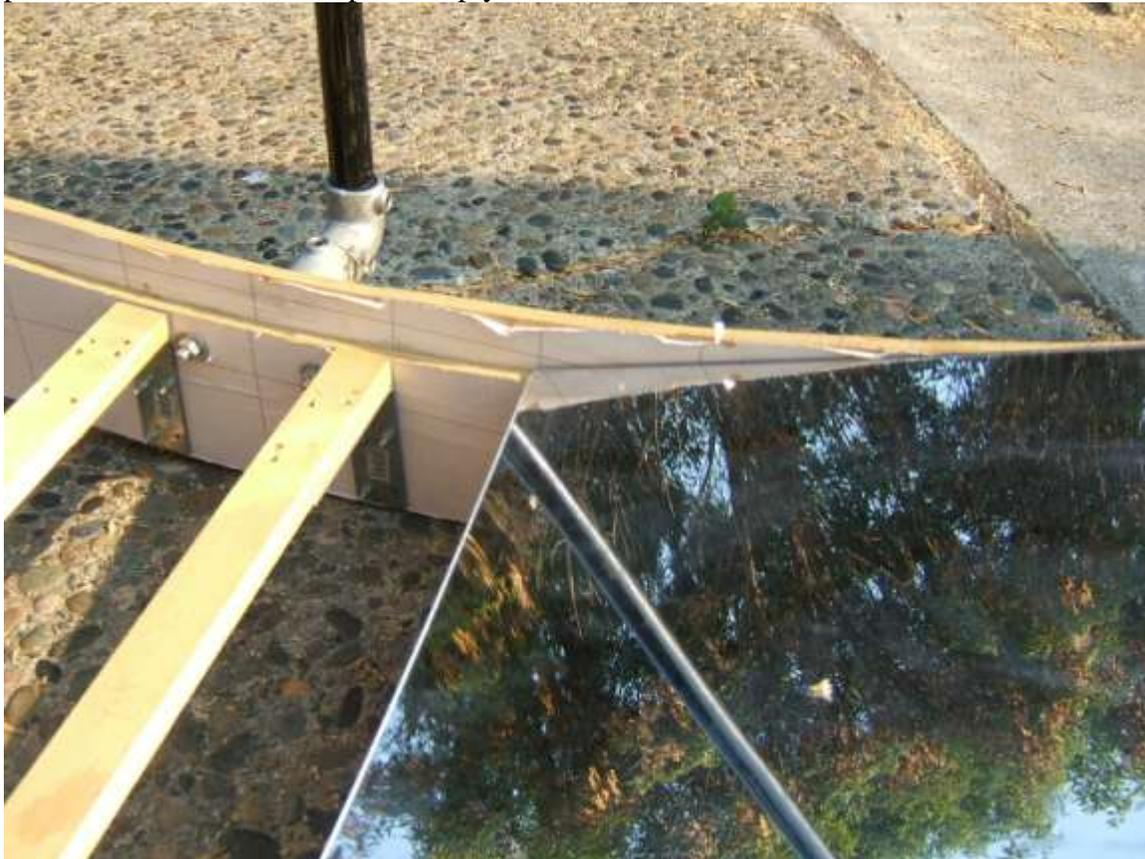
From a single sheet (8' X 4') of ½ inch plywood cut out 4 curves. All four curves follow the equation set forth above. The two “shorter” curves are about 6 inches tall. The two taller curves are about 8 inches tall. Only the top edge of the shorter curve needs to be cut out exactly. This is a miserable painstaking project, but precision here is necessary as a slight distortion can cause the light to entirely miss the cooking surface three feet above.
